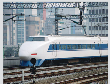
Transportation: Reduce vibration in rail cars and improve track maintenance with pads under rails
