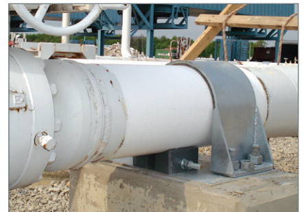
Oil & Gas: Reduce vibration from rotating equipment, as well as thermal expansion on a pipeline
